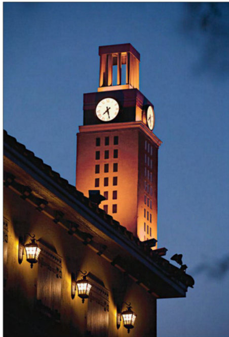
Marc designed the rooftop replica of the University of Texas at Austin Tower. He had the stucco crew mold windows that were then inset with glass tiles. The working clocks are designed to withstand the elements. Marc worked with an electrician to ensure the LED lighting produced a burnt orange recognizable to any Longhorn fan along with other colors.
